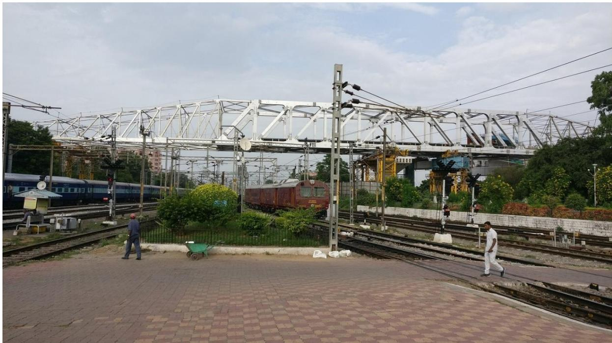
**HMR Oliphenta RoB with dimensions of length 82.6 m, width 17.3m and height 10.55m spanning across 8 existing and 5 future tracks.**
