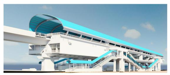
Stations being a window to Hyderabad Metro service are designed to integrate with the urban fabric of the city with minimum visual intrusion into the urban landscape. Typically a station is located above the road and consists of four levels, namely, Street, Concourse, Platform and Roof.
