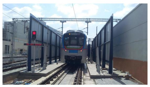
Fig:-7 - Automatic Train Wash Plant
